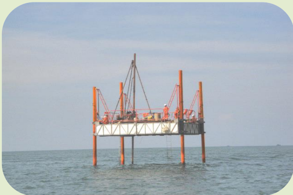
Offshore investigation on Jack-up Platform
