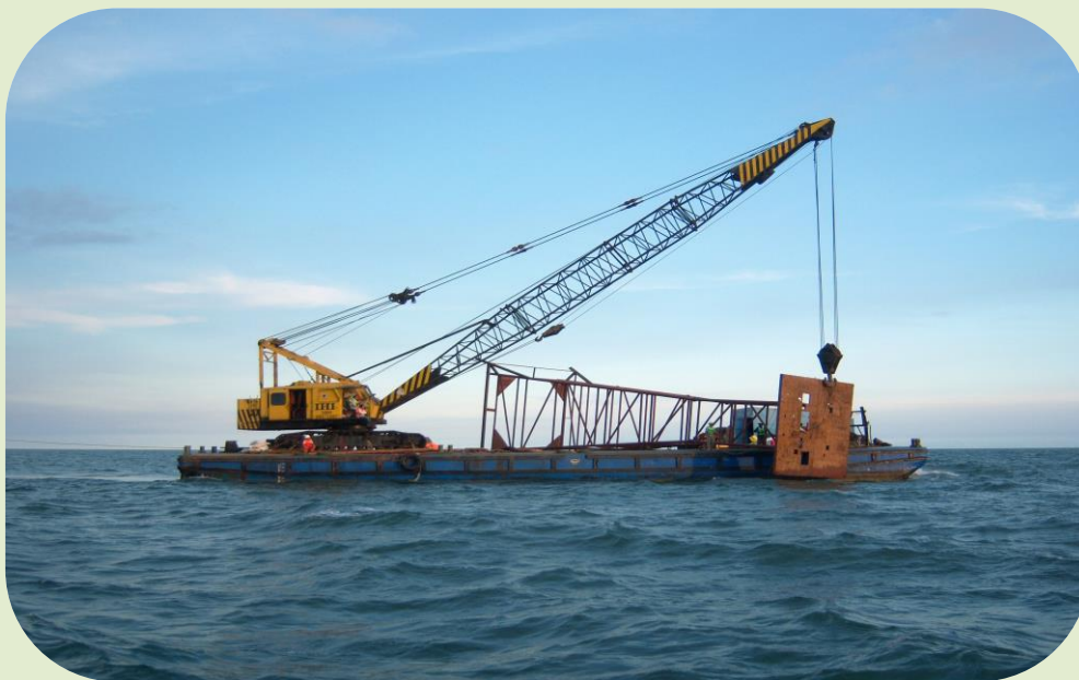
Offshore investigation on fixed Platform
